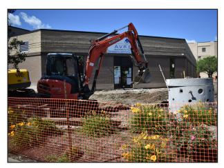
Above: An excavator removes old pavement to make way for new sidewalks and blacktop. Construction will be managed by Fahs Construction Group.
